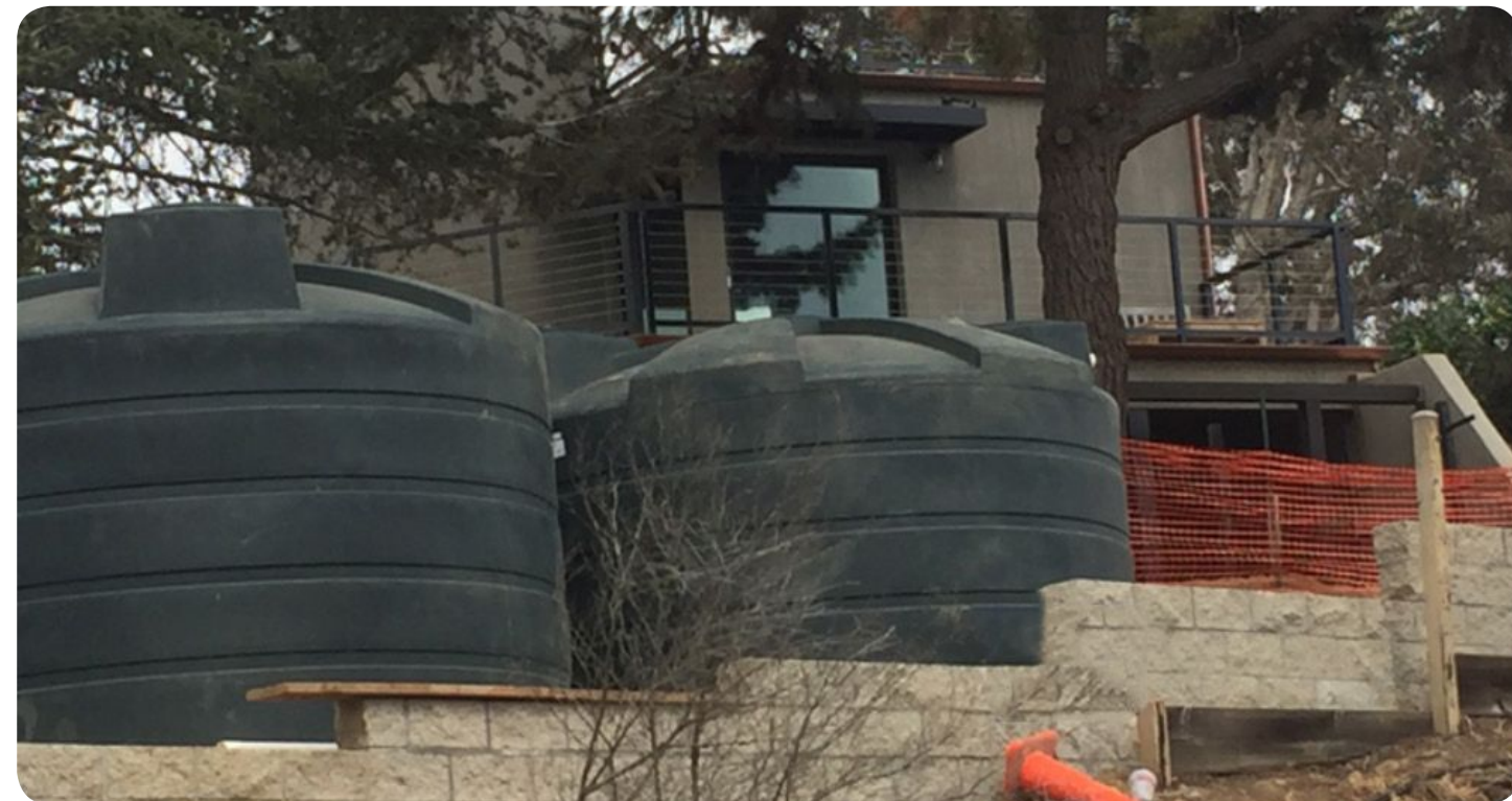
Figure 13: Installation of Two 5,000 Gallon Cisterns
